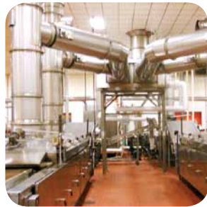
Energy Recovery Heat Exchanger installation
