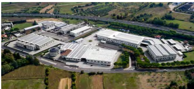
CEIA S.p.A. headquarters, Vicinaggio, Arezzo [Italy]
